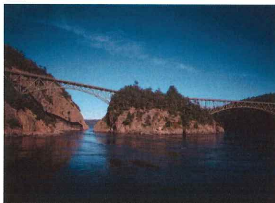
写真-70 Pass 島と Deception Pass Bridge
